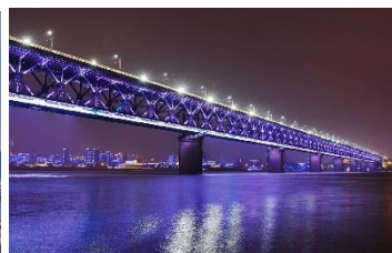
Yangtze River Bridge
